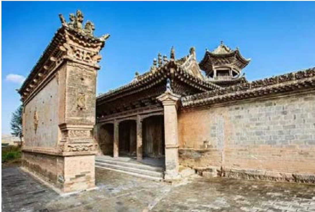
Figure 15. Screen wall of Hongshuiquan Mosque
