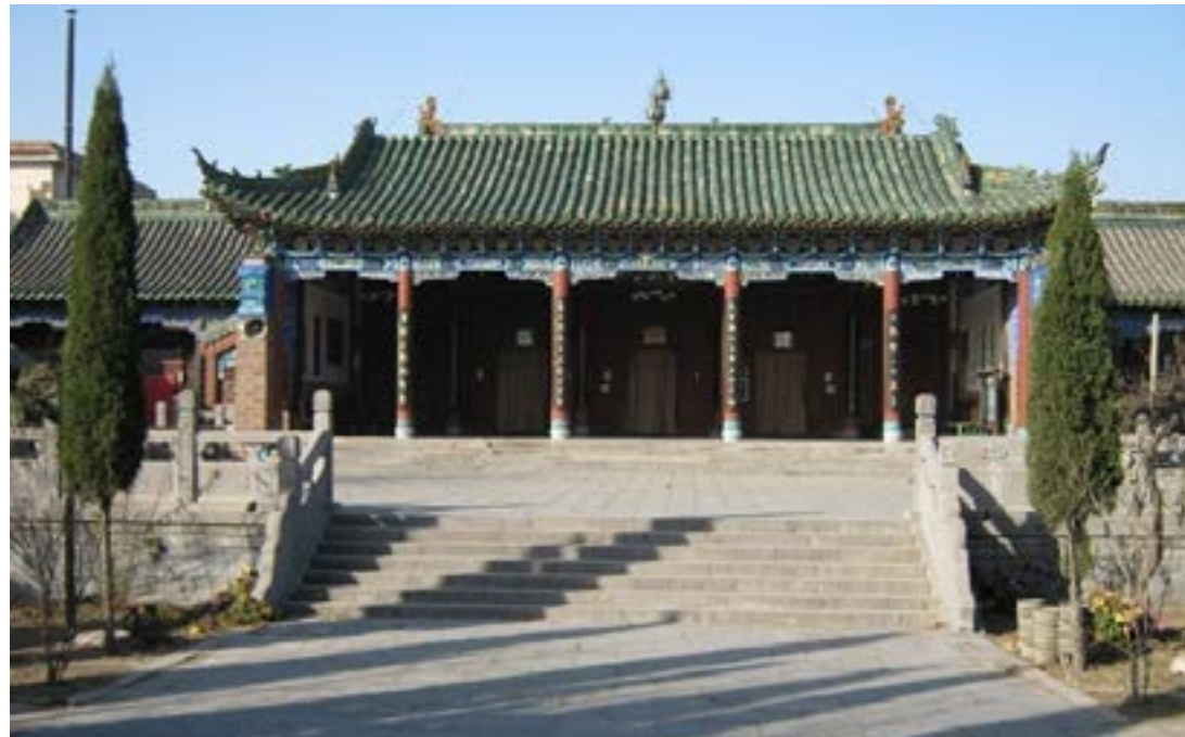
Figure 6. Moon platform and step units of East Great Mosque, Kaifeng
